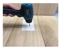
2. Open hollow spot by drilling, if necessary make additional drillings
