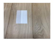
1. Locate hollow spot and mask drilling spot
